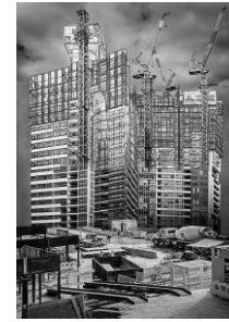
Under construction v6 Entry Graeme James
